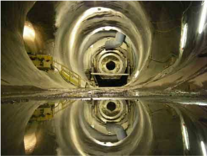
Shell construction of the Gotthard Base Tunnel
